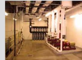
The mechanical system was transformed into a high-performance low-energy consumption system by incorporating a ground source heat pump geothermal exchange. Utilizing the earth as a heat source (in the winter) or a heat sink (in the summer) will boost efficiency and reduce the operational costs of heating and cooling systems. To reduce heat gain on affected facades, perimeter insulation was enhanced and windows were reframed and glazed to reduce air conditioning loads.
