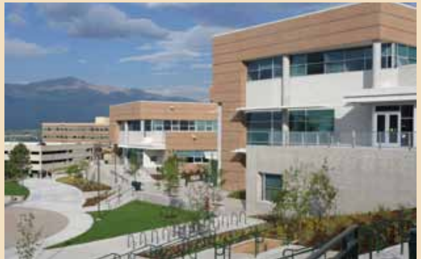
University of Colorado Colorado Springs, Osborne Center for Engineering and Science
