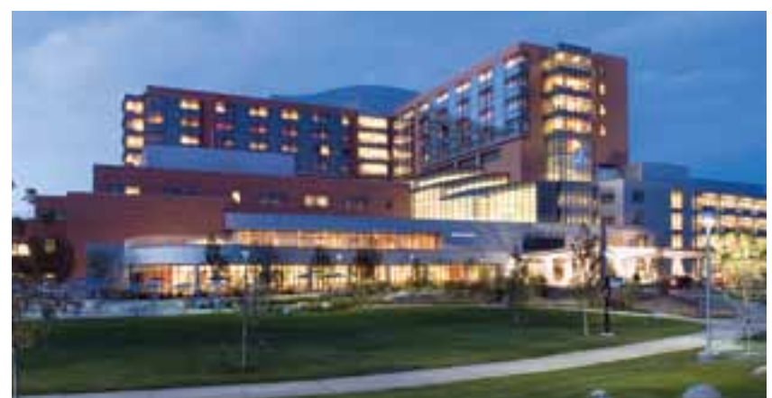
Children’s Hospital Colorado Aurora, Colorado
