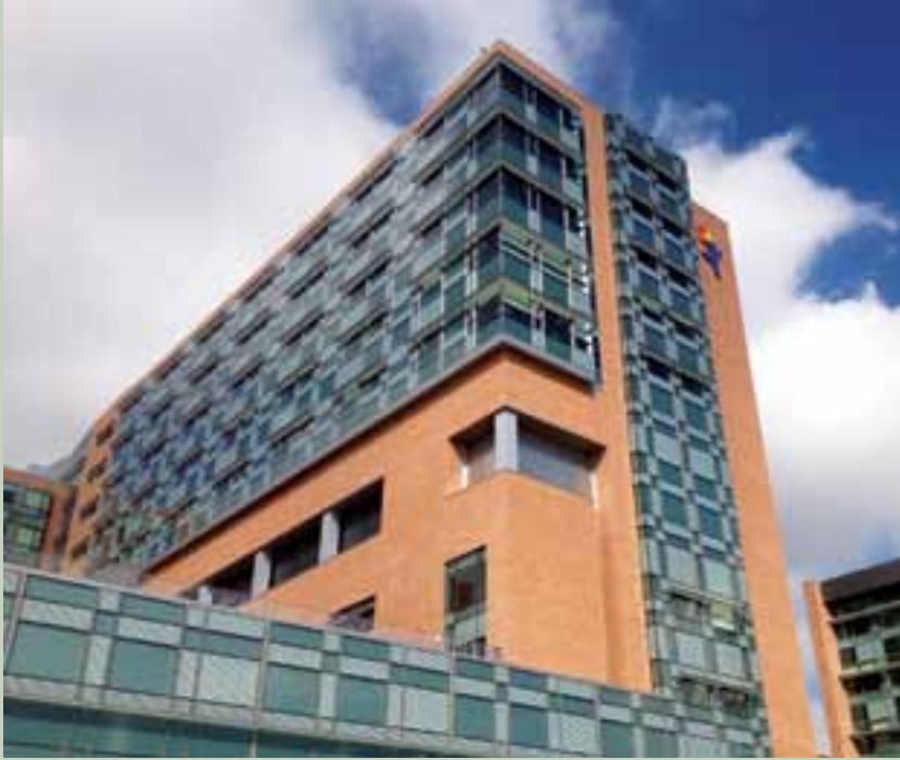
Children's Hospital Colorado East Tower addition and renovations
